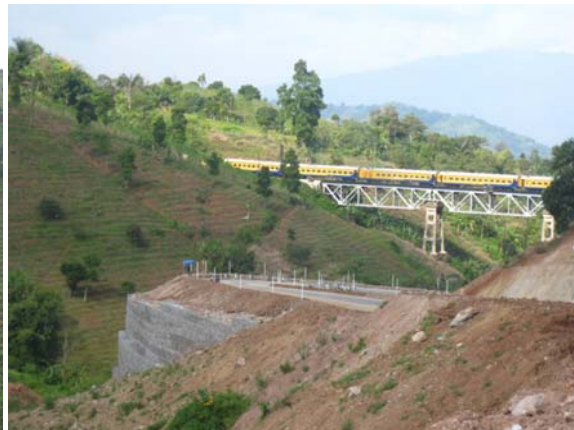
1 st Trial Phases (STA 3+200)
