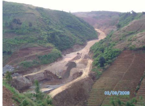
Foundation Preparation (STA 2+800)
