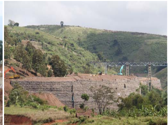
1 st Trial Phases (STA 4+000)
