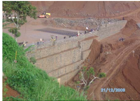
Construction Progress 40 % (STA 2+800)
