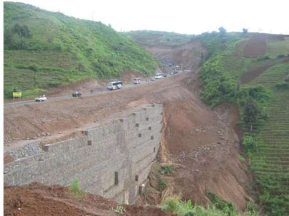
1 st Trial Phases (STA 2+800)
