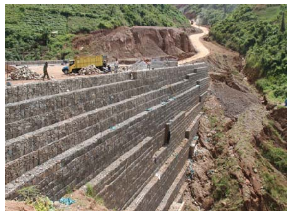
Construction Progress 80 % (STA 2+800)
